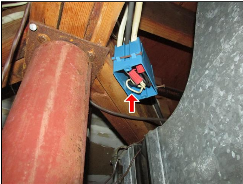
7.3 Item 4(Picture) Missing cover plates.
