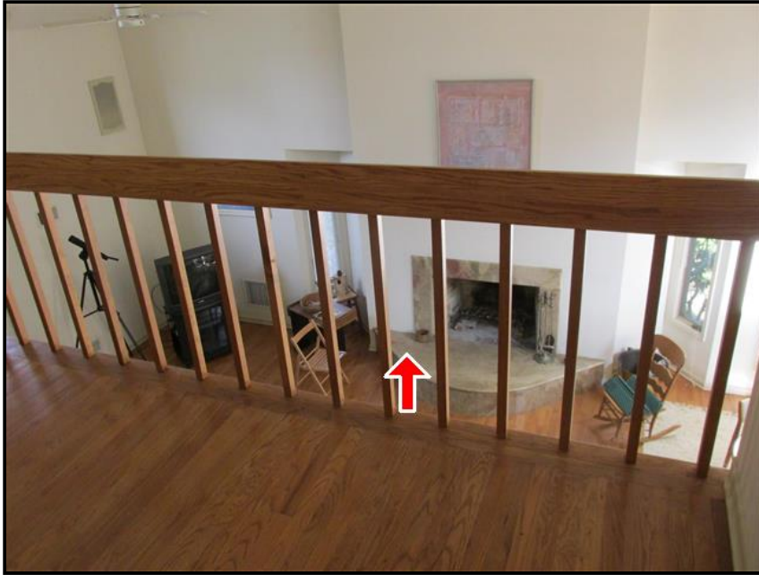
4.3 Item 1(Picture) Spindles spaced to far apart.
