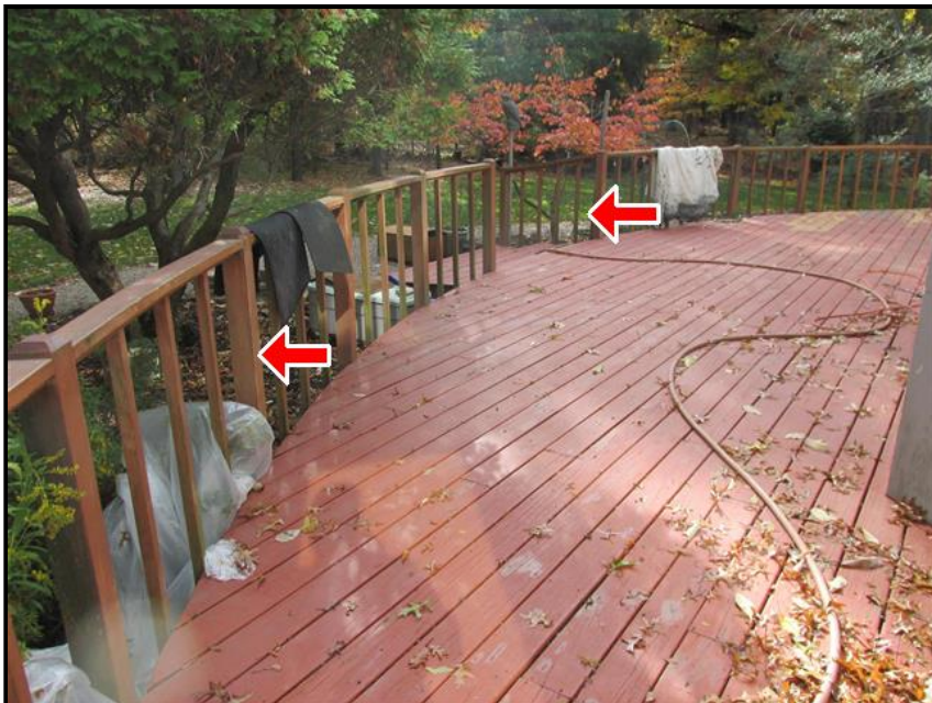
2.3 Item 3(Picture) Deck spindles spaced to far apart.
