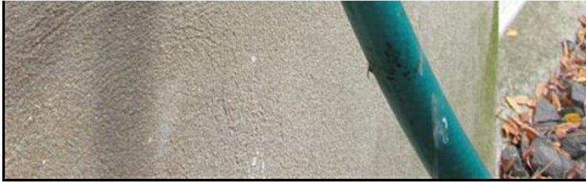
6.1 Item 1(Picture) Hose bib handle leaks.
